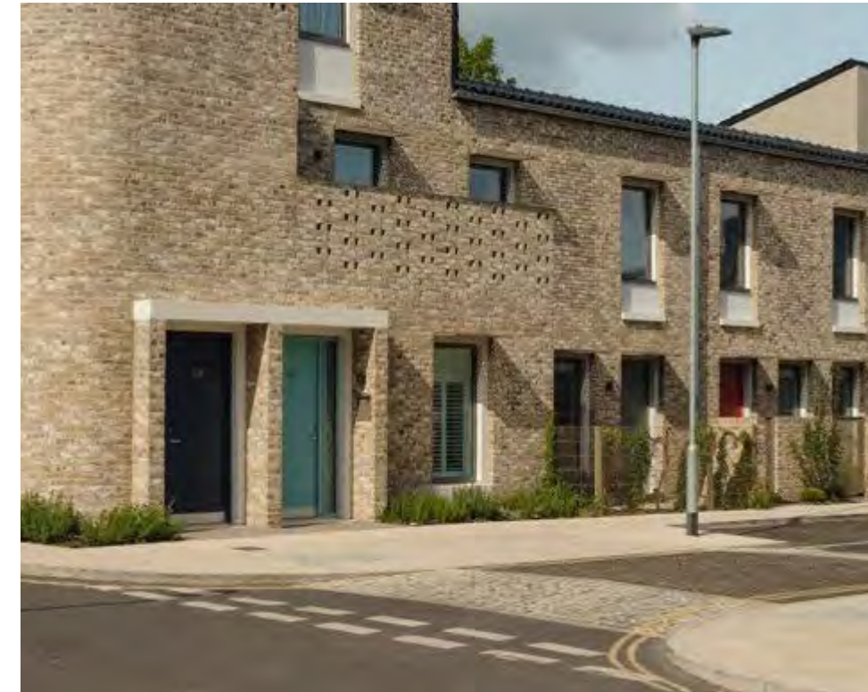
Clearly visible entrances with defined points of entry. Goldsmith Street, Norwich- Mikhail Architects
