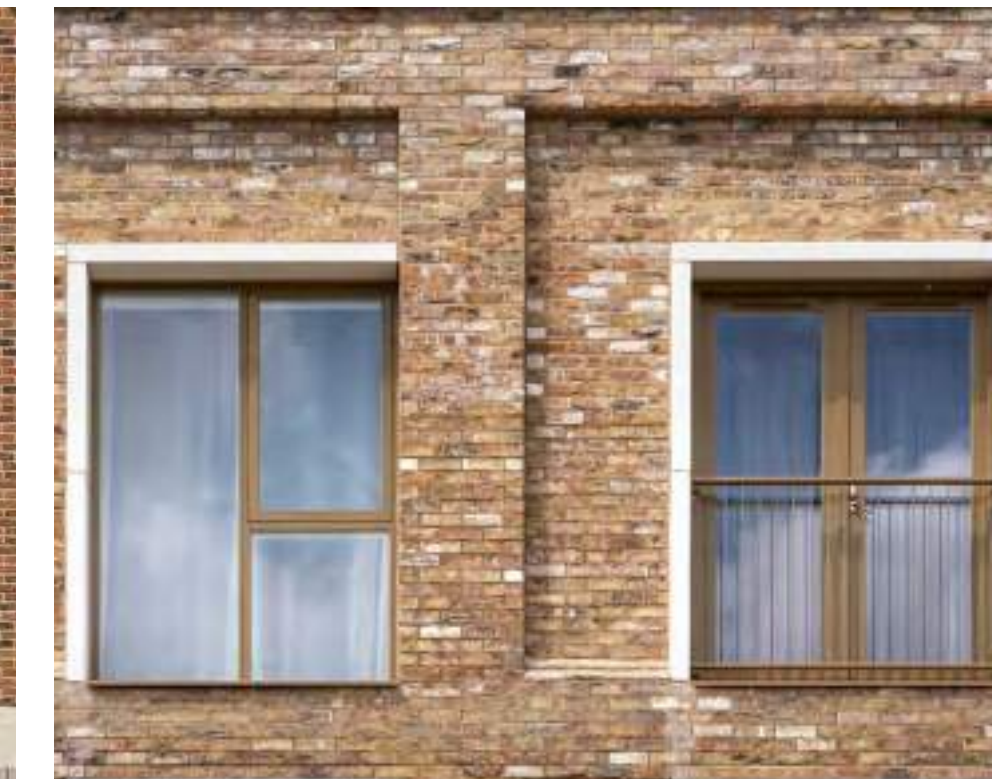
Use of complimentary materials for detailing. West Green Place, London - HTA Design
