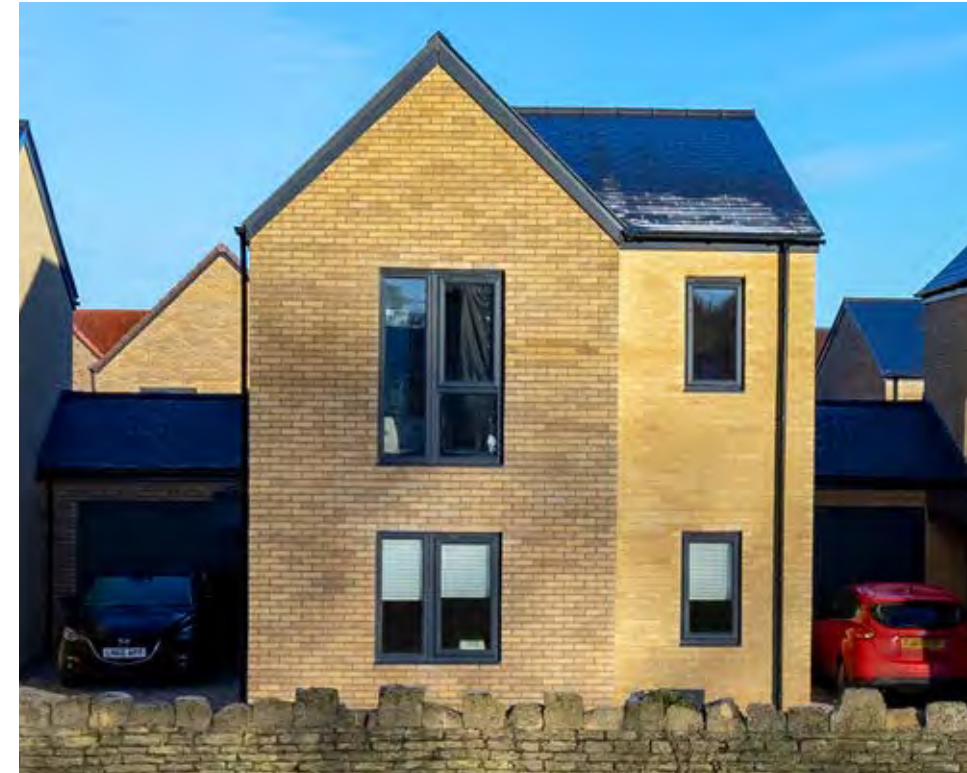
Clear and consistent placement of doors and windows. Mulberry Park, HTA Design LLP
