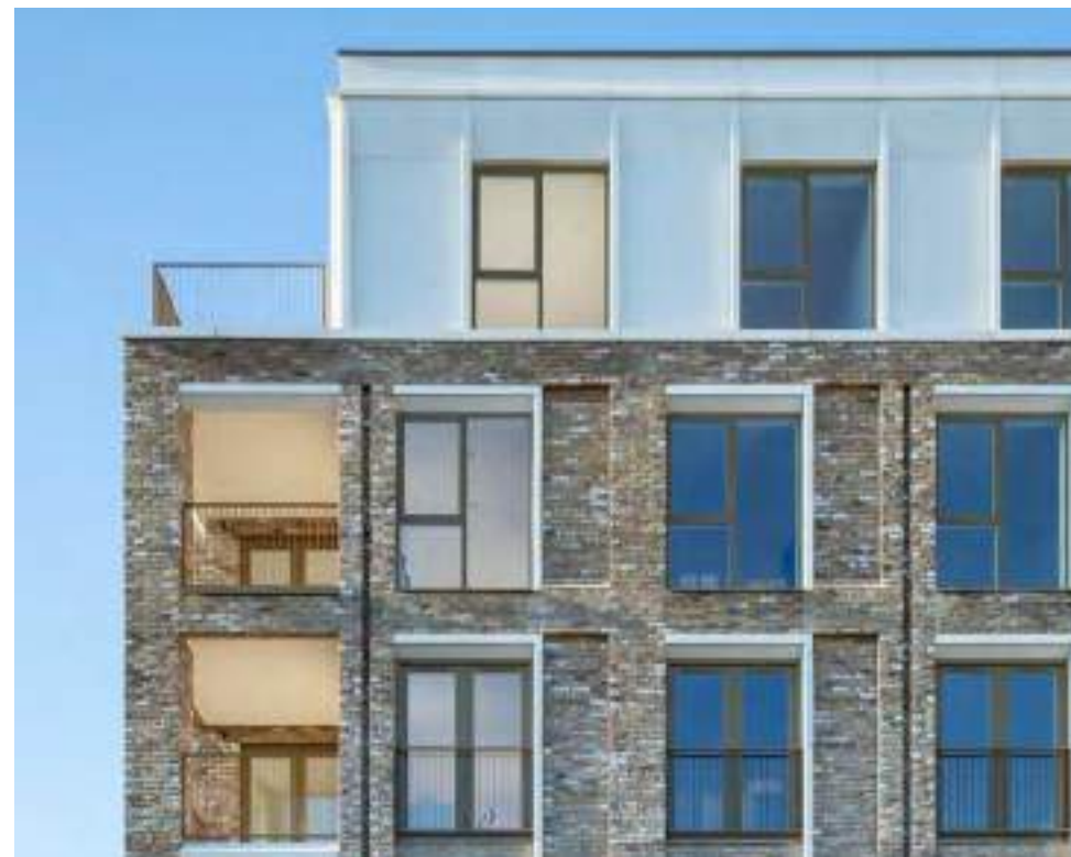
Recessed roof articulation for the apartment blocks. West Green Place, London - HTA Design
