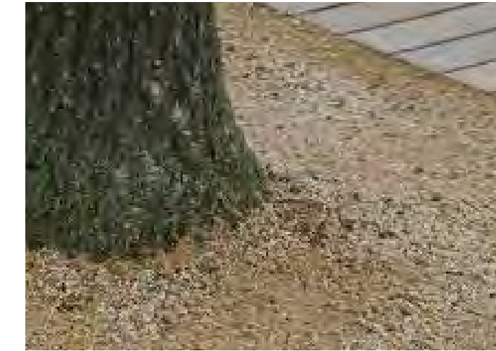
Consolidated/self-binding gravel to tree pits
