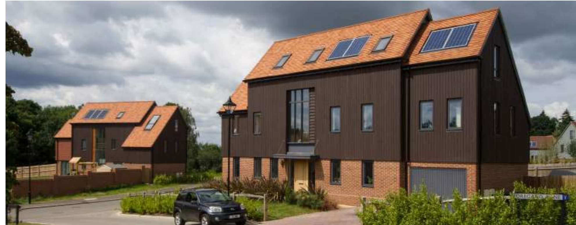
Dark brick tones must be used as the predominant material, as shown above. Roofs must be predominantly plain clay tiles. Leithfield Park, Surrey - HTA Design
