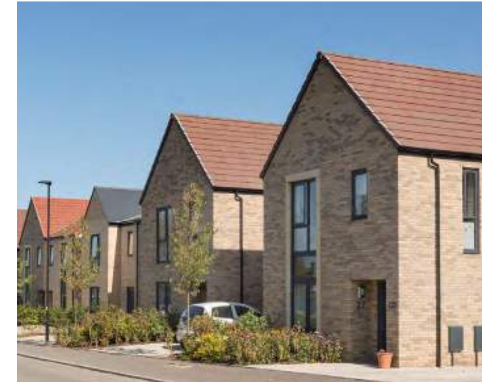
Frontage includes elements of soft landscape, in addition to well-designed hardscape. Mulberry Park, Bath - HTA Design LLP
