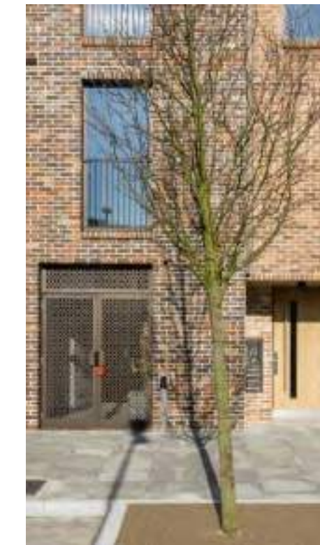
Use of architectural detailing and materials to differentiate entrances from service and storage access.
