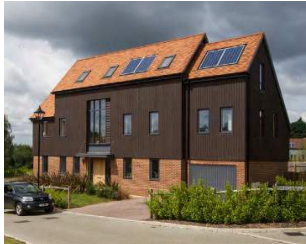
The predominant design articulation must feature a datum line, where brick bases are paired with weatherboarding elements for upper floors. Leithfield Park, Surrey - HTA Design
