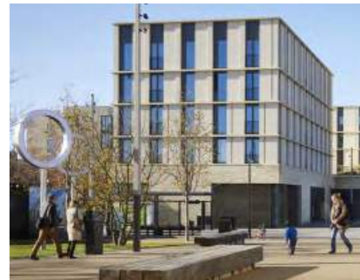
Large windows that maximise internal light. North-west Cambridge Business Park - Stanton Williams Architects
