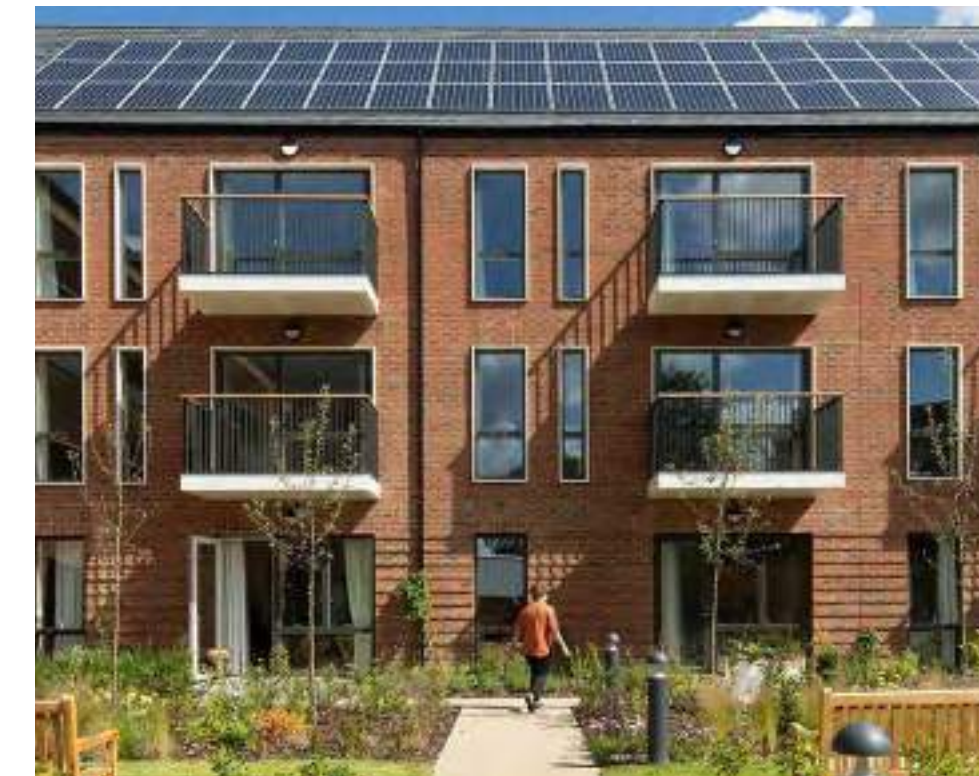
Larger openings to capture long views within Dunton Fanns. Ansell Court, London. PRP Architects.
