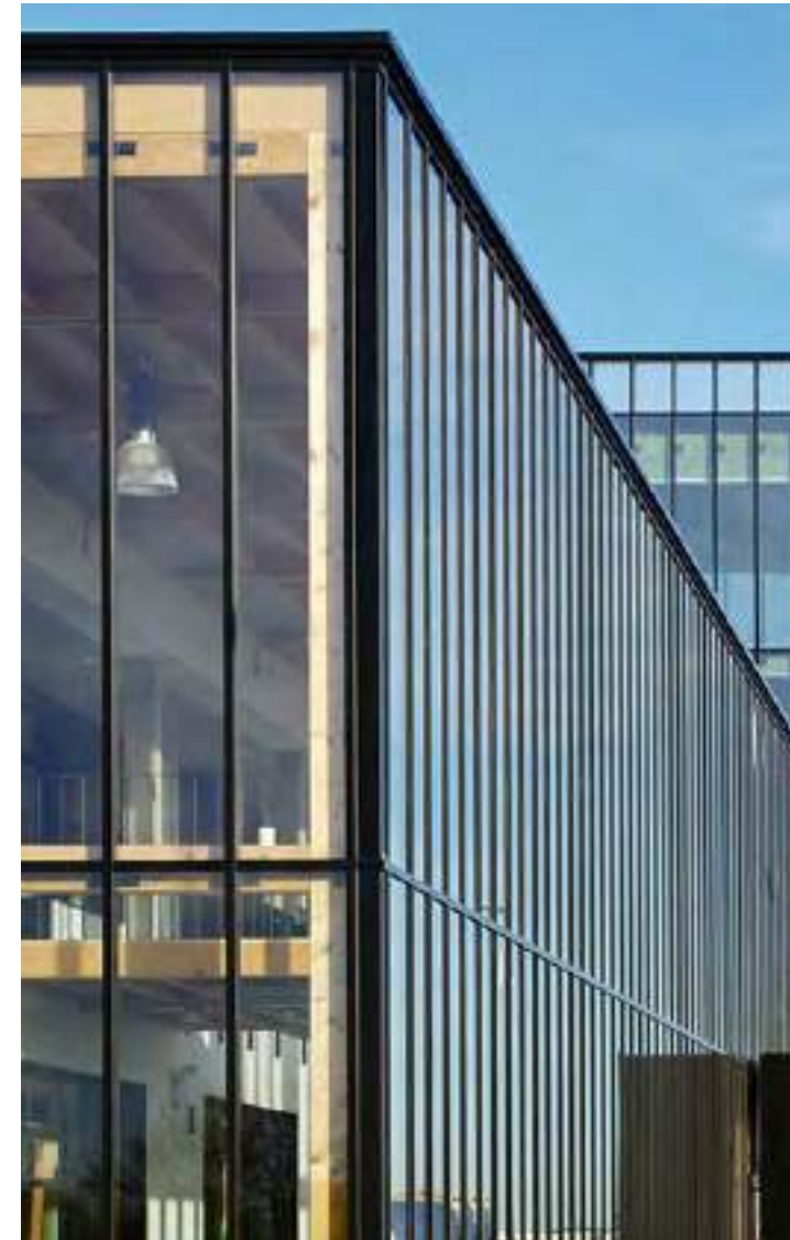
Emphasis on verticality with the use of curtain walls. Alconbury Incubator - AHMM Architects
