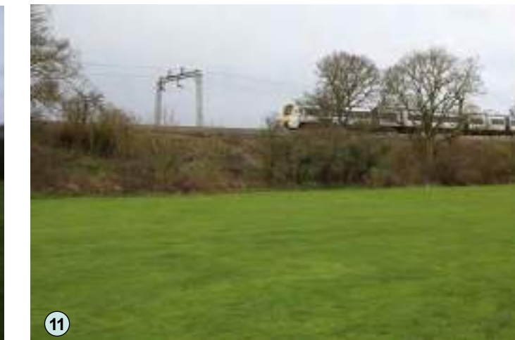
View of the Rail Lines
