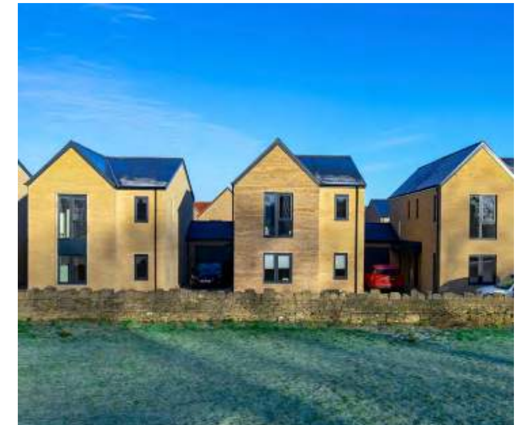
Continuity in the roof profile. Mulberry Park, HTA Design LLP.
