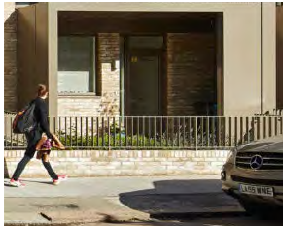
Use of landscape and boundary treatments to create continuous frontage. Ely Court, London- Alison Brooks
