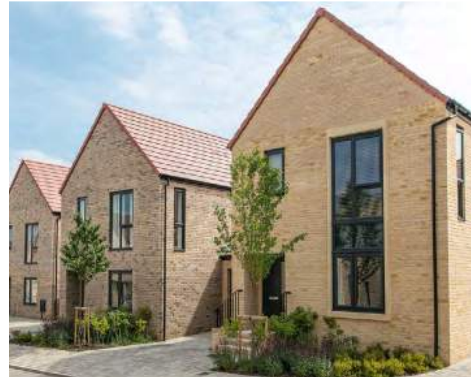
Use of materials demonstrating the design rationale and use to distinguish key architectural elements. Mulberry Park, HTA Design LLP.
