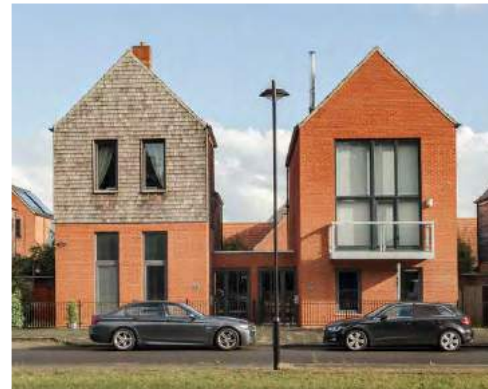
Elevations of groups of houses must create a coherent street elevation in terms of building proportions, materials, roofing and placement of doors and windows. Upton, Site C, Northampton. HTA Design LLP.
