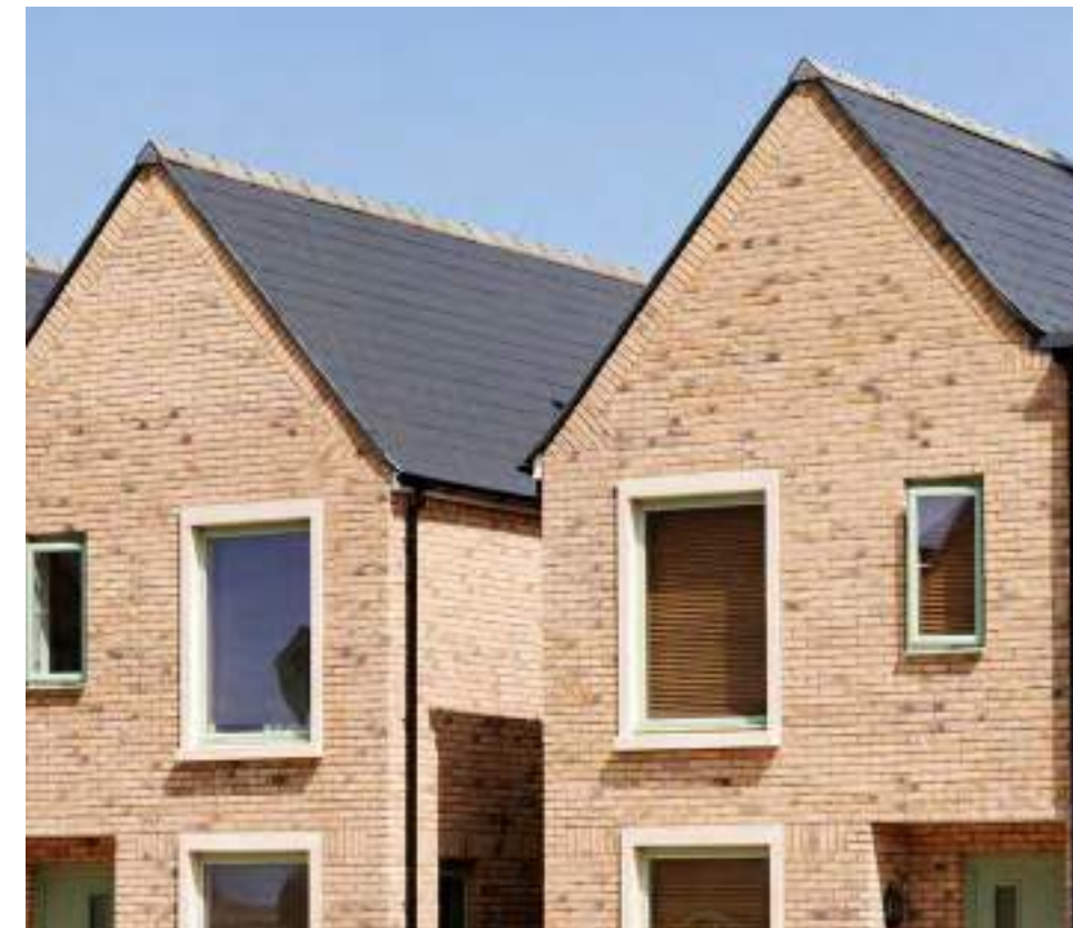
Highlighting on windows with white, light beige or grey tones of detailing. Castle Court, Portland - HTA Design
