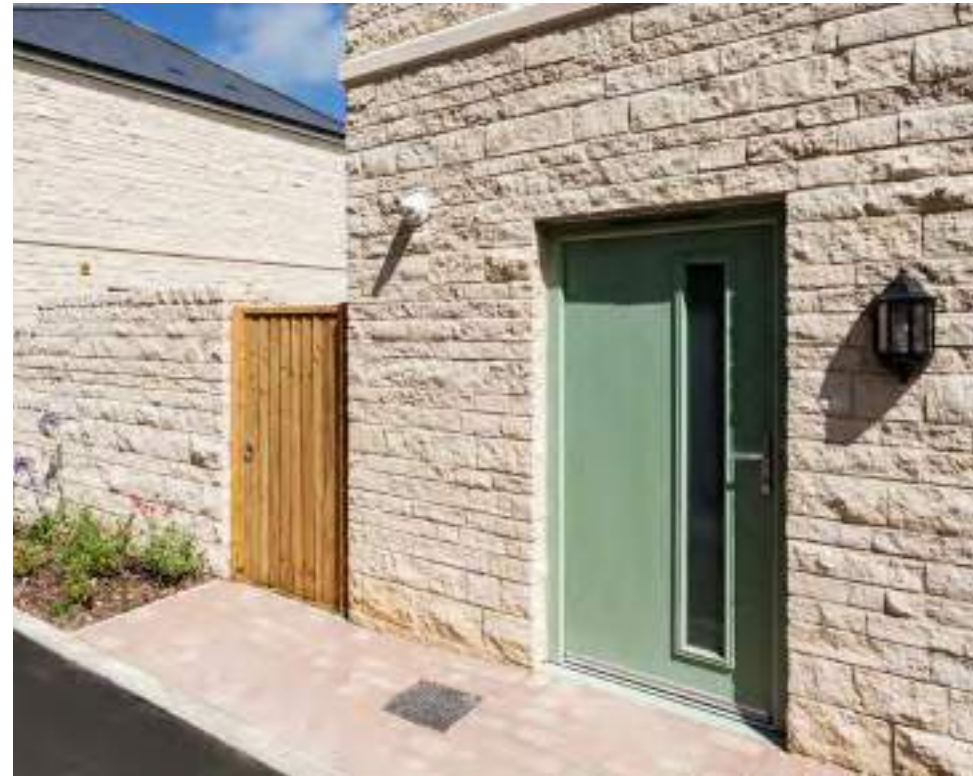
Clearly visible entrances with defined points of entry. Castle Court, Portland - HTA Design
