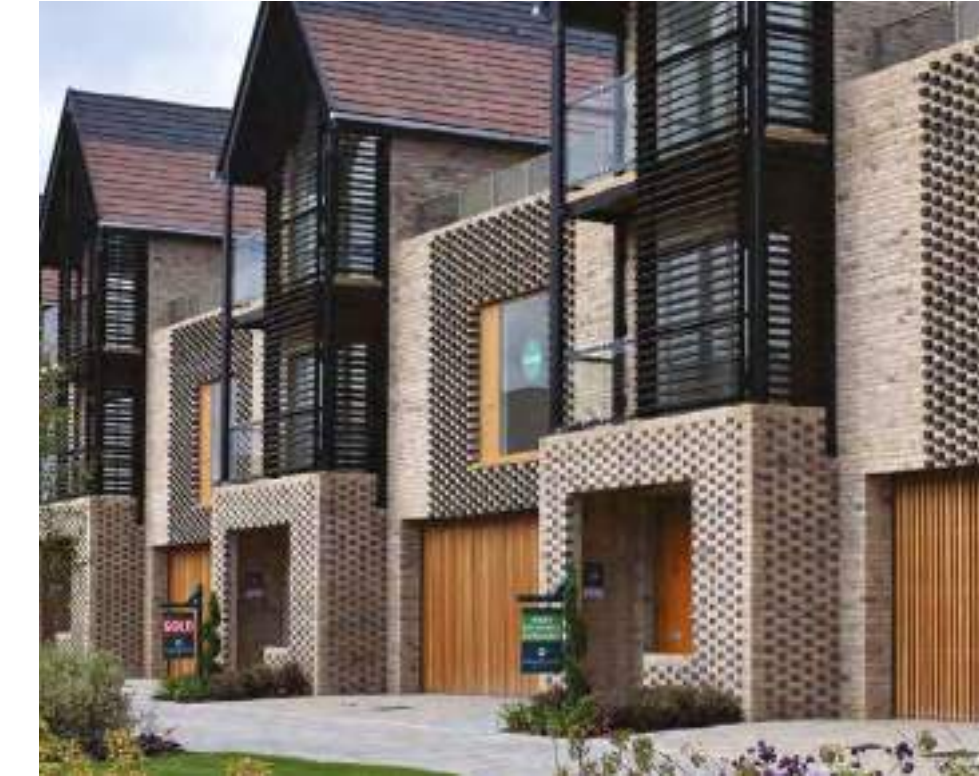
Double height articulation could be used to reinforce vertical expression. Adelaide Wharf, London. AHMM Architects
