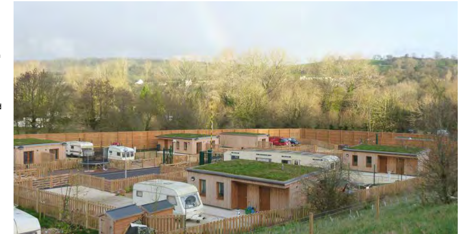
The layout of the site allowing safe and well designed access. Bristol Road Traveller Site, Bath
