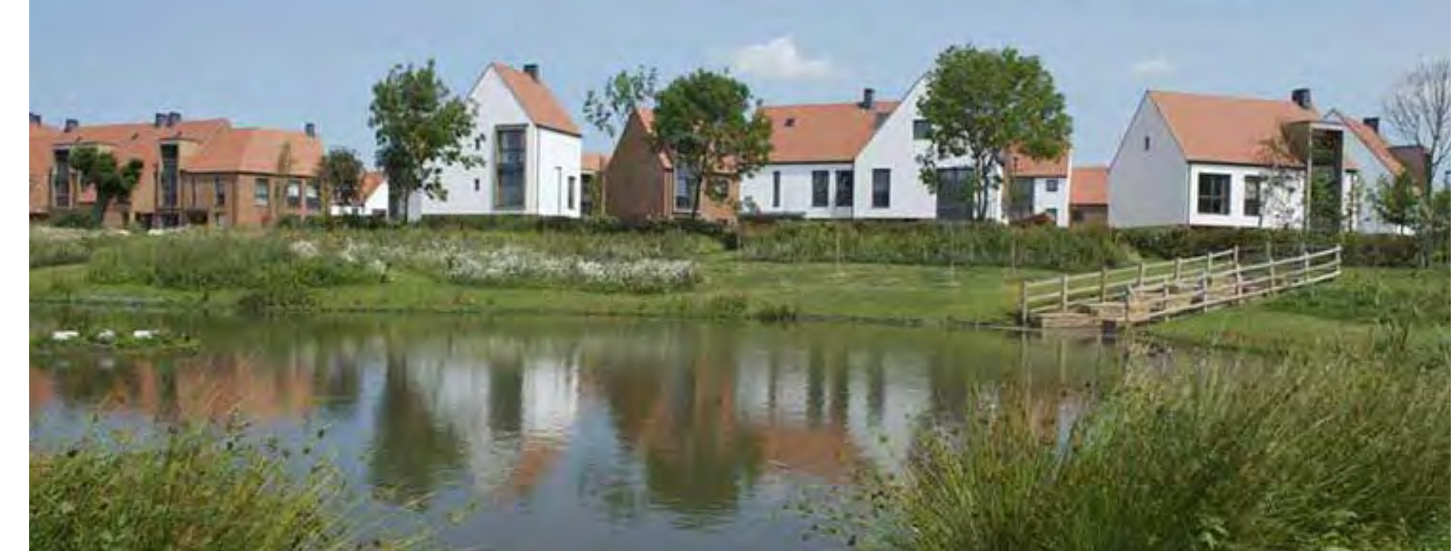
Variations in roof profiles to add variety and to respond to the intended character of Dunton Waters. Derwenthorpe, York - JRHT
