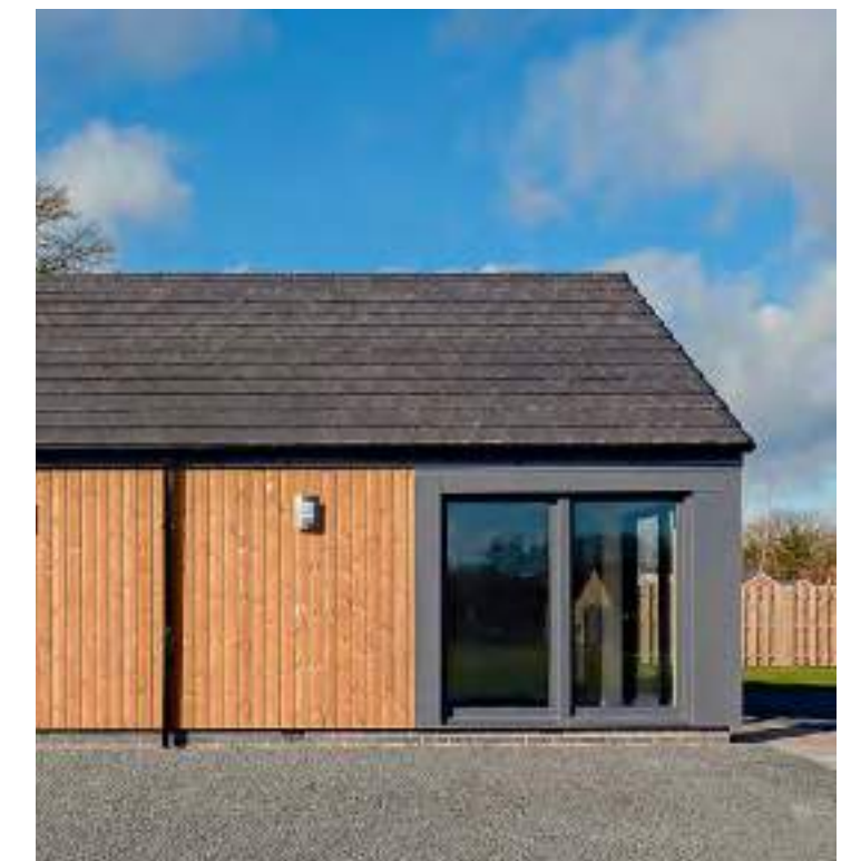
Day room materiality. Old Damson Lane
