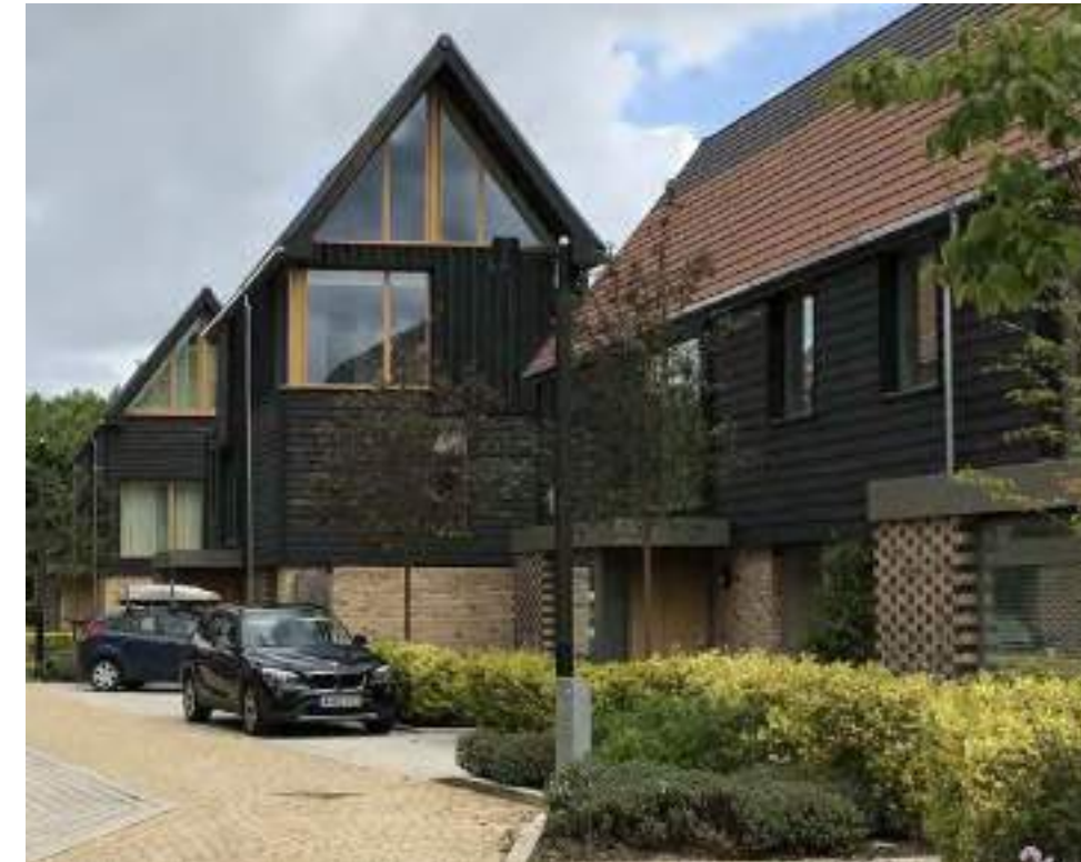
Elevations must be designed to positively contribute to the street environment and to the Dunton Woods character. Abode, Cambridge
