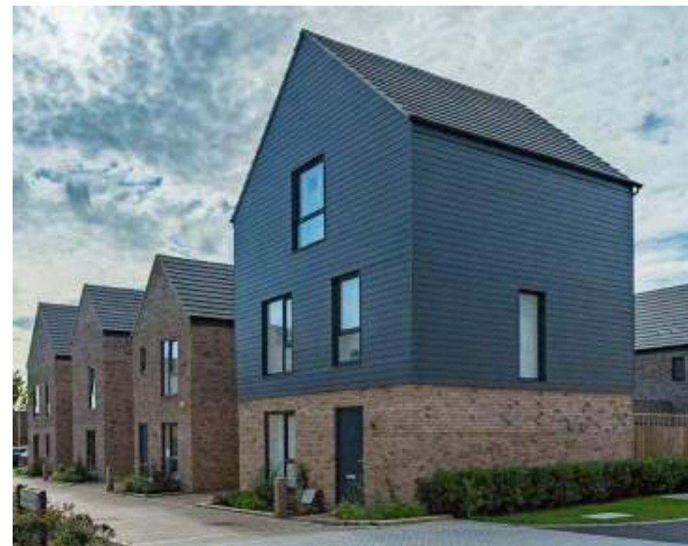
The use of complimentary materials, such as weatherboarding timber cladding which sits upon a brick plinth is encouraged. Cheshunt School - HTA Design
