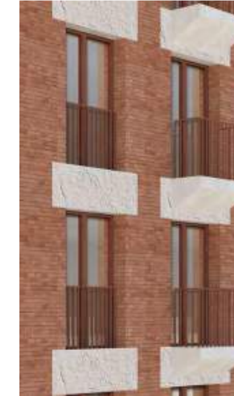
Recessed balcony design with metal balustrade detailing. Winstanley and York Road Estate, London - HTA Design
