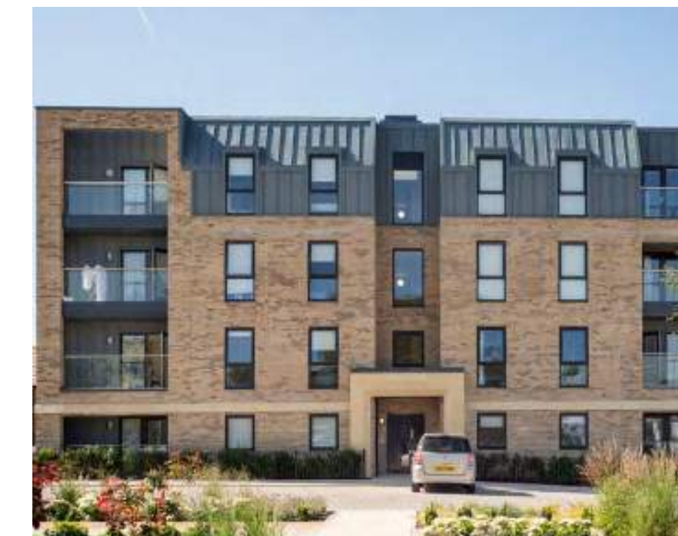
Use of varied material to emphasize on entrance to apartments. Mulberry Park, Bath - HTA Design
