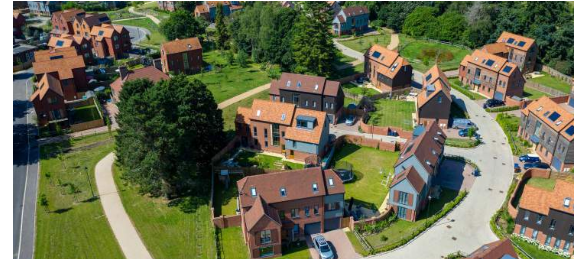
Roofs of adjacent buildings (even when varying in shape) must be designed together so they form a composition in terms of their type, scale, pitch, orientation and projecting elements. Leithfield Park, Surrey - HTA Design
