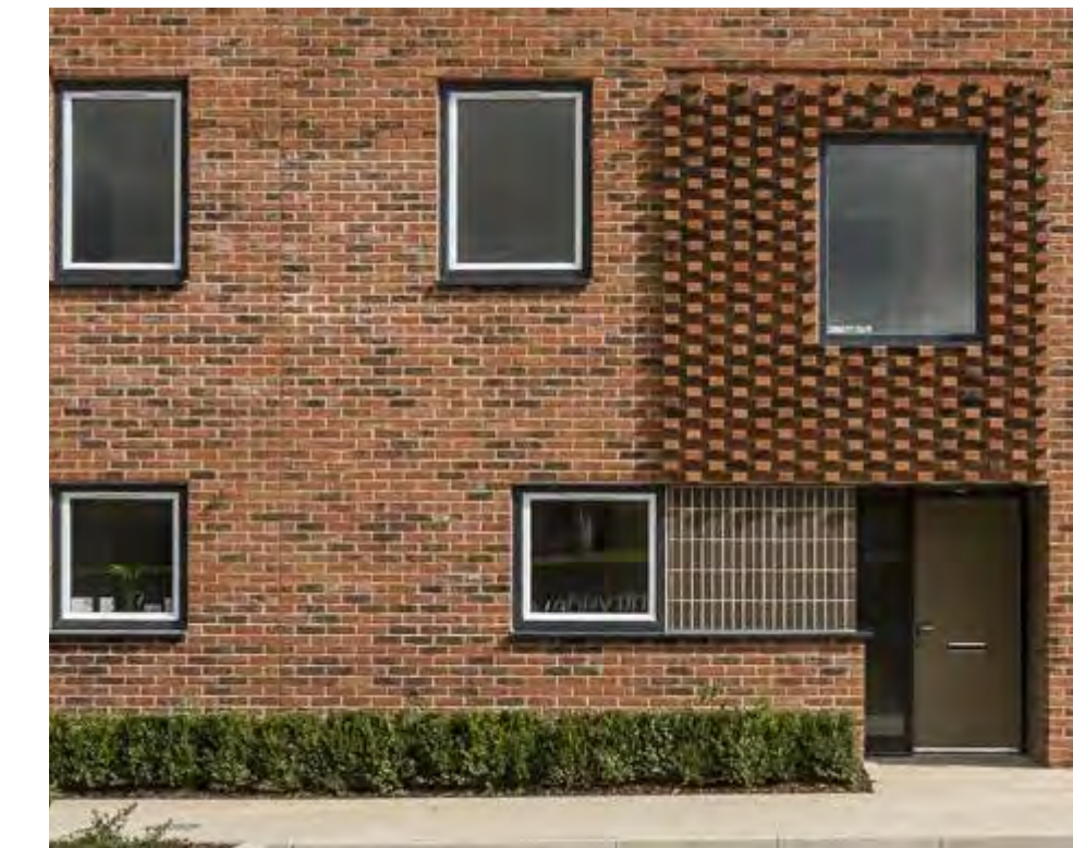
Tone of red brick at the primary material. Horsted Park, Kent - Proctor & Matthews
