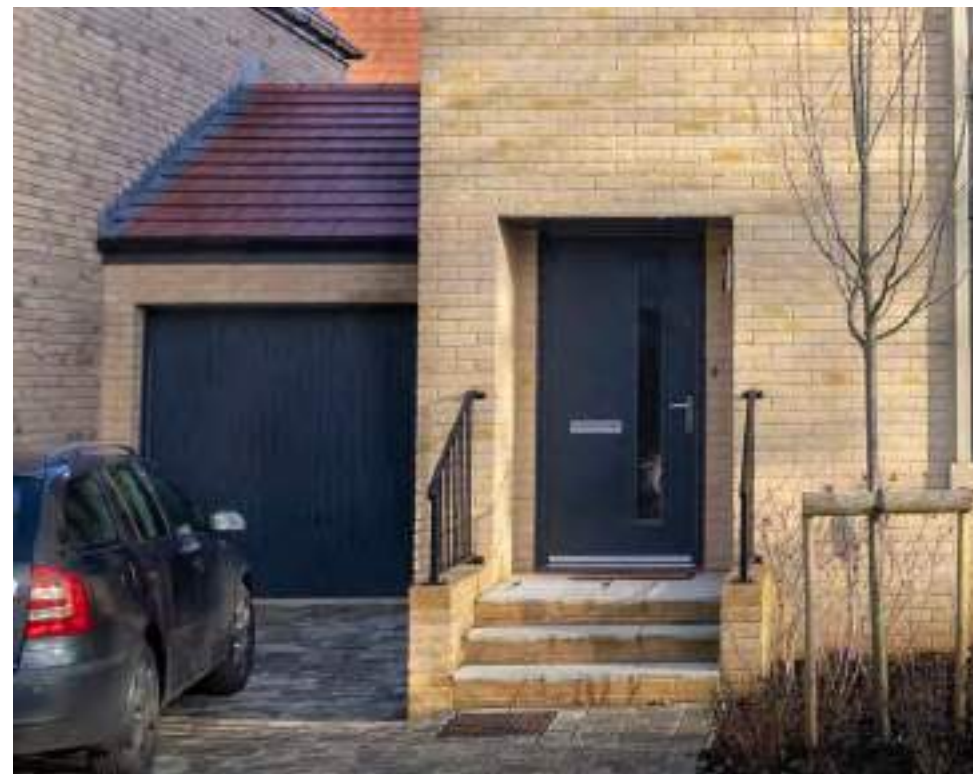
Recessed zones to further emphasize entryways. Mulberry Park, Bath - HTA Design LLP
