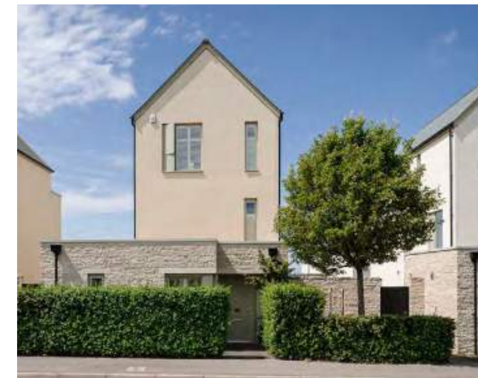
Clear definition of private and public zones; within planting within the private zone. Osprey Quay, Portland - HTA Design LLP
