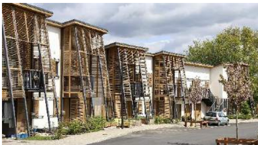
Ex. 1: Hanham Hall, South Gloucestershire, HTA Design LLP – homes with modern wood shading
