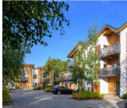
Hanham Hall, South Gloucestershire, HTA Design LLP
