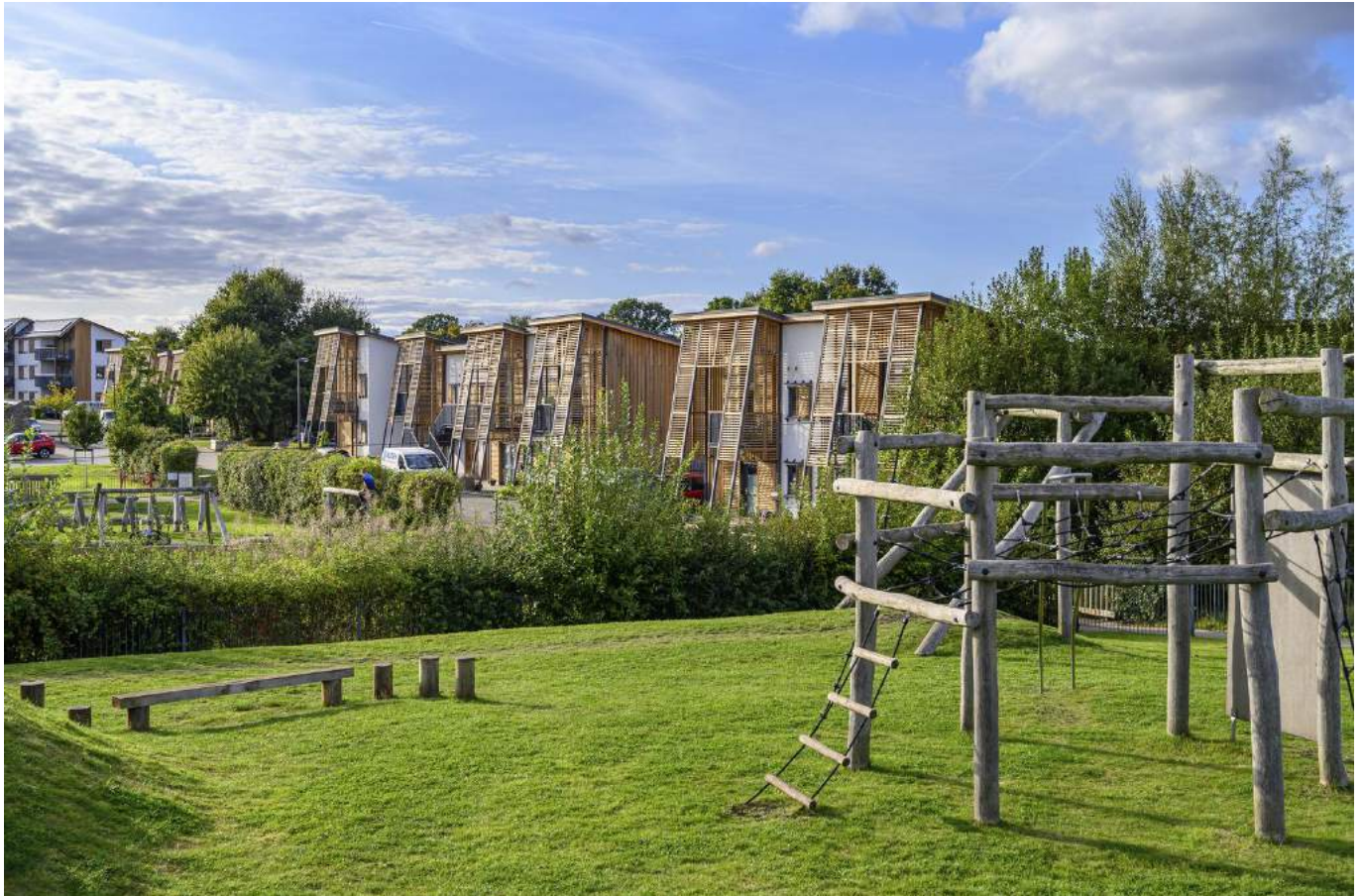
Figure 4: Hanham Hall, South Gloucestershire – HTA Design LLP
