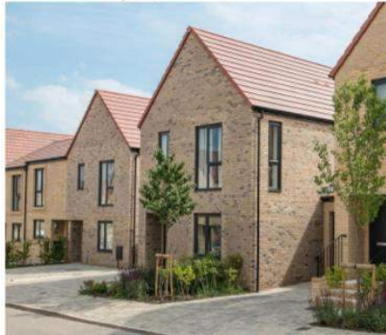
Ex. 1: Mulberry Park, Bath, HTA Design LLP – traditional homes with brick and pitched roofs
