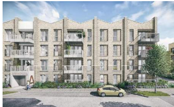
Ex. 2: Southall Waterside Phase C, Ealing HTA Design LLP – flats with traditional brick work but with balconies and pitched roofs
