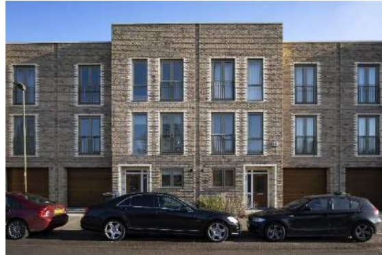
Ex. 2: Trinity Square, Barnet, HTA Design LLP – flats with traditional brick work
