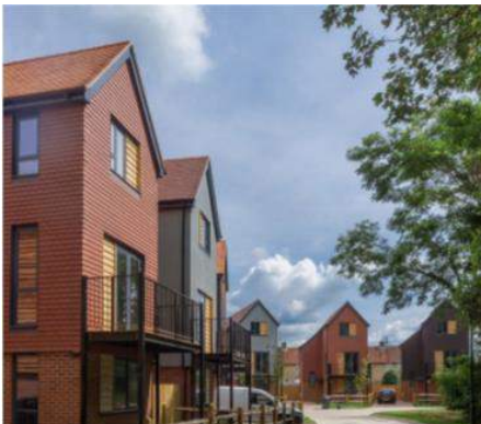
Ex. 1: Milford Hospital, Surrey, HTA Design LLP – traditional homes with balconies and modern materials
