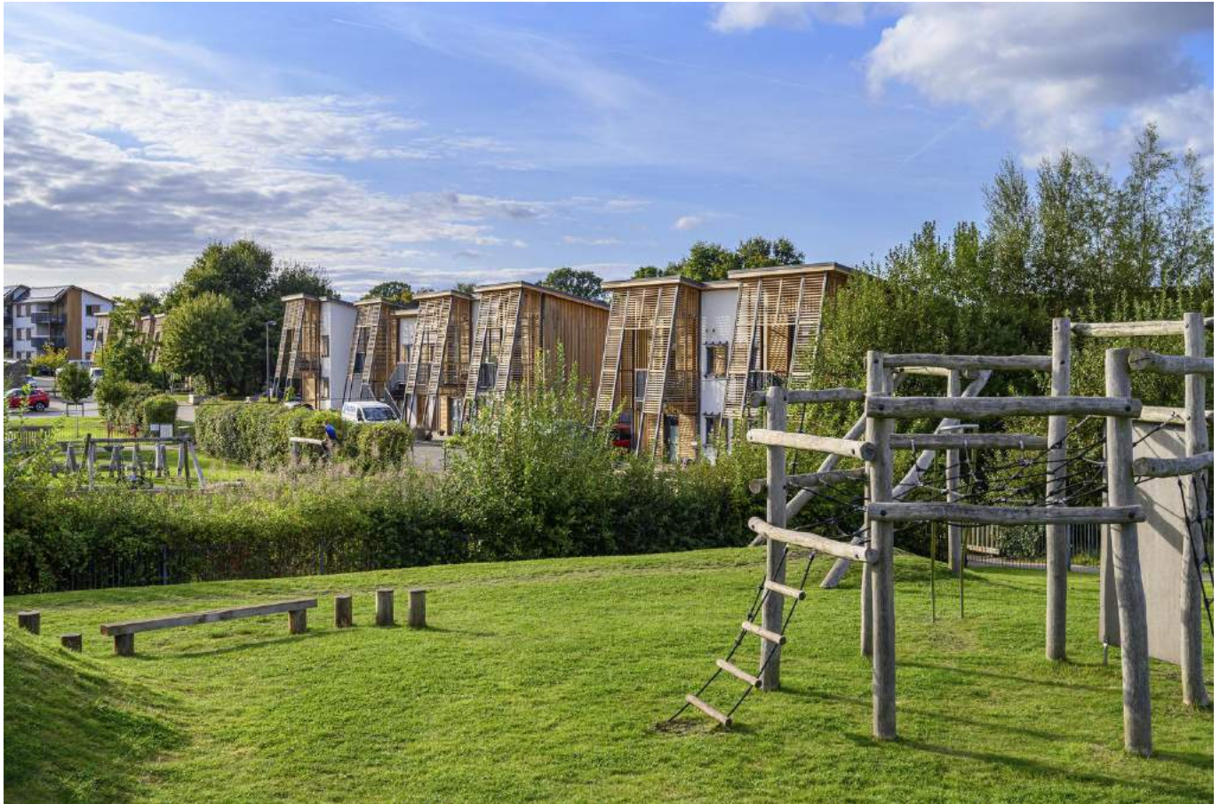
Figure 3: Hanham Hall, South Gloucestershire – HTA Design LLP
