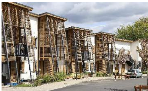
Ex. 1: Hanham Hall, South Gloucestershire, HTA Design LLP – homes with modern wood shading
