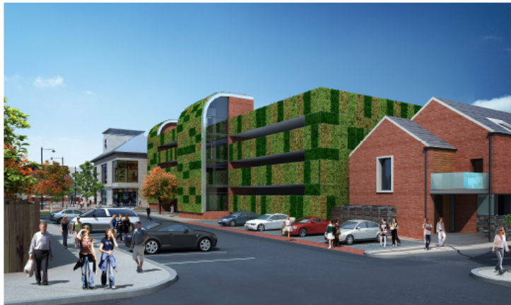
Perspective 06: Residential Building 'D' in foreground with Building 'B' (Carpark) + Building 'A' behind; looking South along North Service Road
