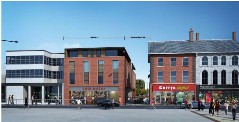
Perspective 02: Building 'C' (Link) in foreground with Building 'B' (Carpark) + Building 'A' behind; looking Northwards
