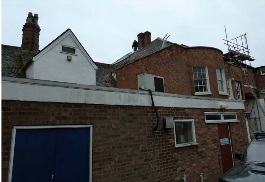
Modern single storey extension to rear of gabled stair tower
