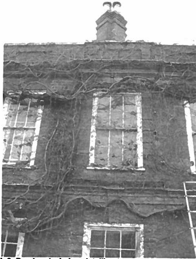
Photograph 3: Dominant window detailing to second window from east end
