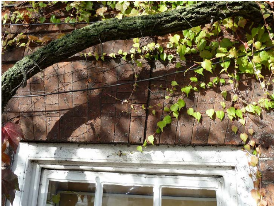
Rubbed brick lintel and keystone
