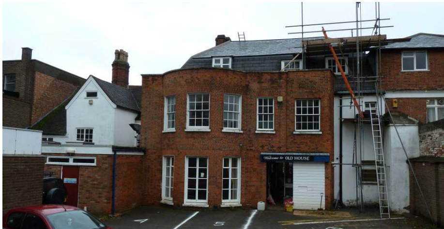
Modern extension and stair tower (left) with curved bay of western rear elevation.
