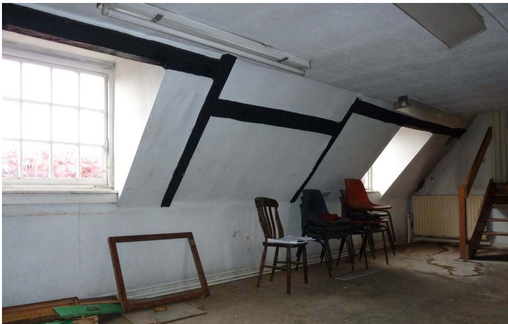
Joggled butt side purlin roof structure
