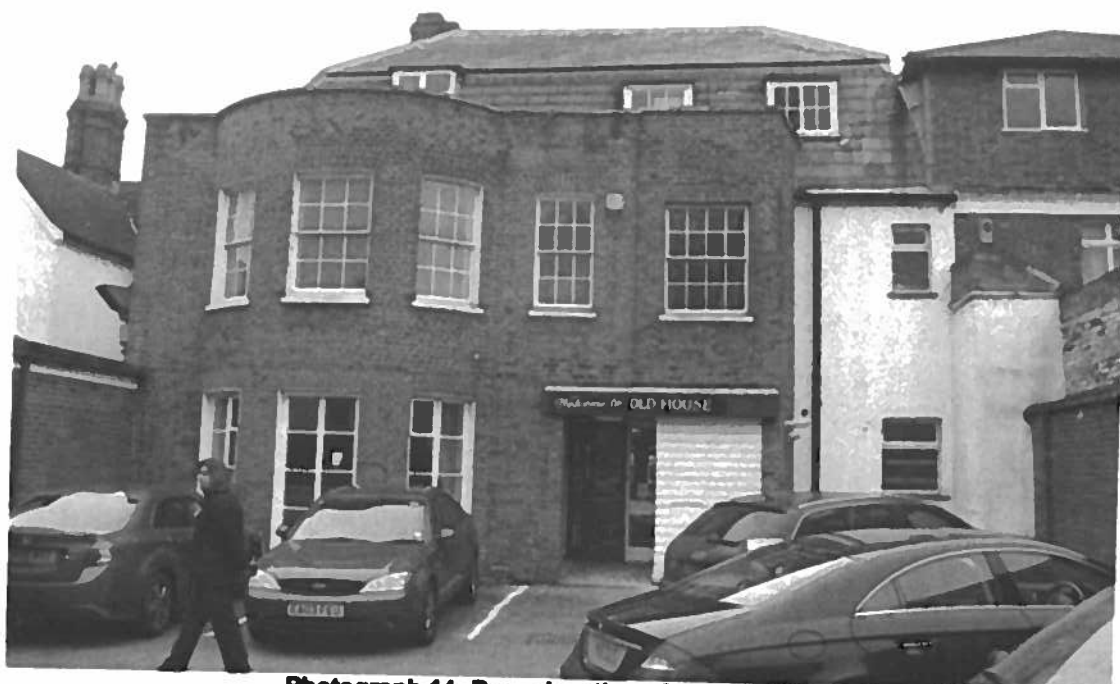
Photograph 14: Rear elevation of west building
