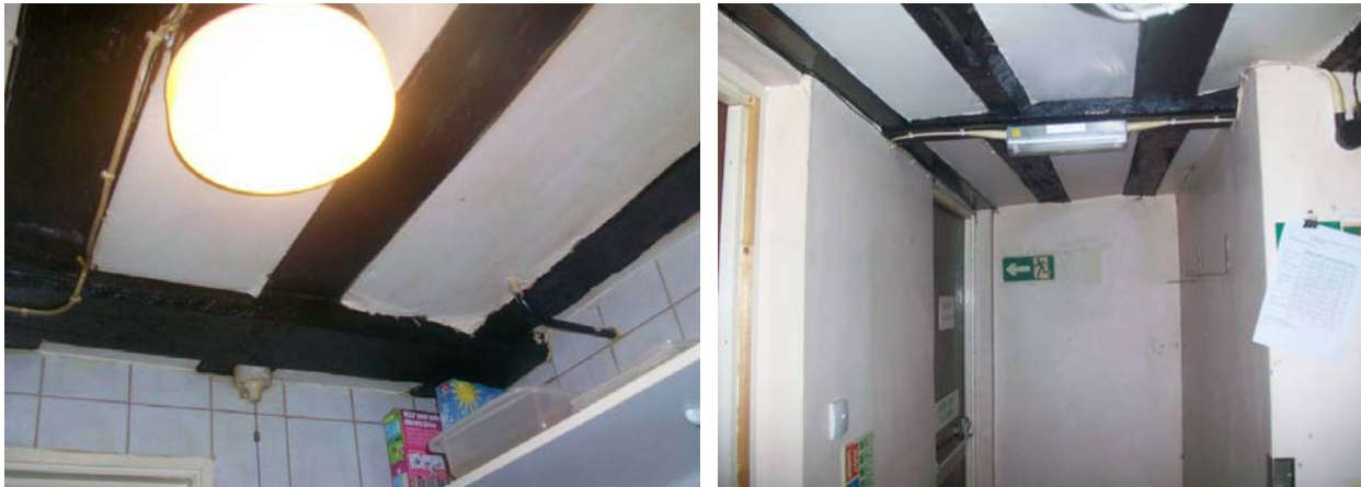
Left: Ground floor kitchen ceiling - beam and joists.
