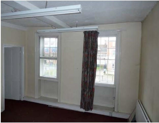
Room 2 – Left: Two sashes with secondary glazing Right: Detail of sash and shutter moulding
