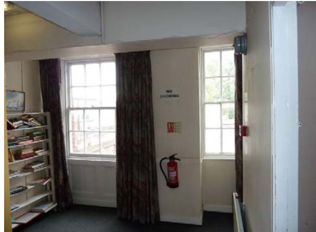
Left: Room 3 – One sash in curved bay – One sash adjacent to bay with secondary glazing
