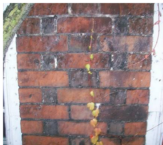
Penny struck pointing, flared headers and queen closers to both front and rear elevations
