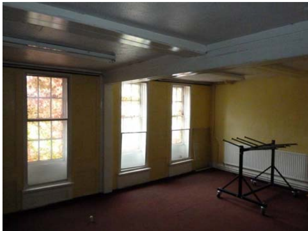
Left: Room 4 – Three (of four) sashes – Binding joist probably supported by RSJ
