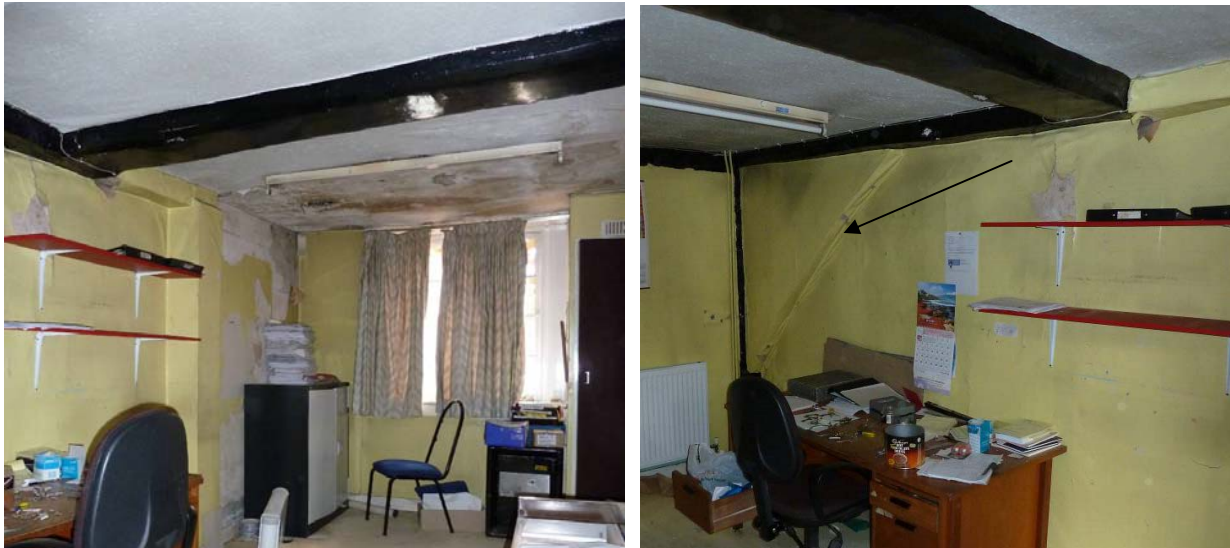
Room 7 (office) - Above left: Looking towards Shenfield Road
