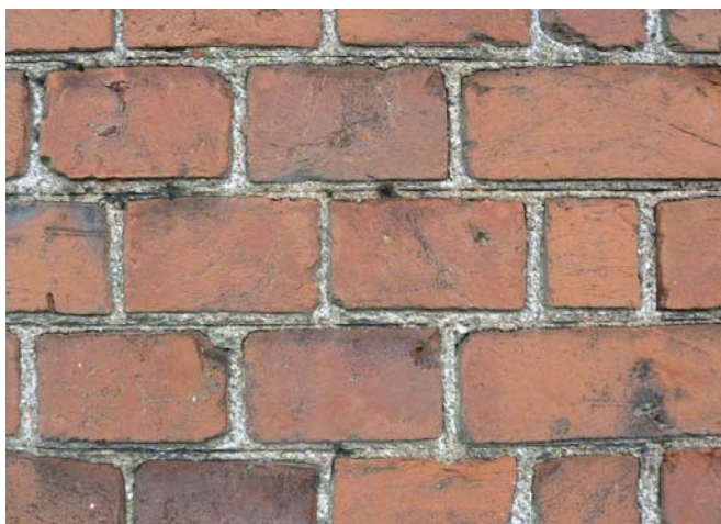
Penny struck pointing, flared headers and queen closers to both front and rear elevations
