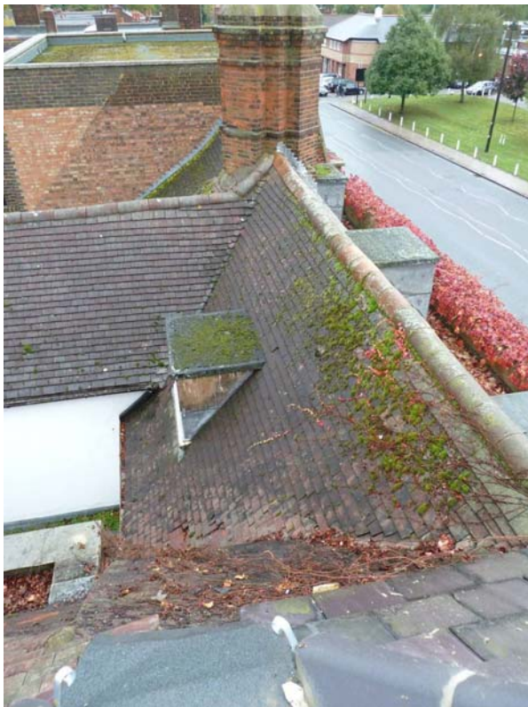
Left: Peg tile roof of eastern building.
