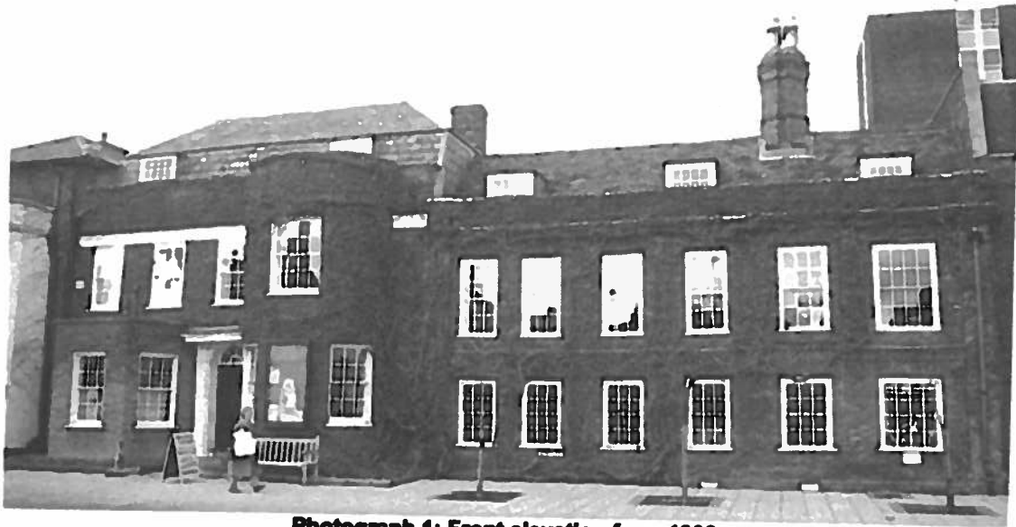
Photograph 1: Front elevation from 1990
