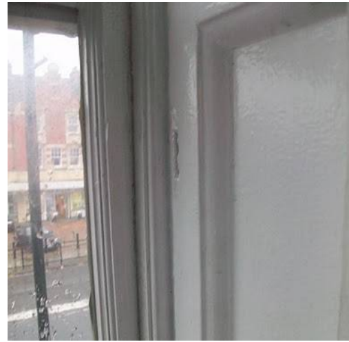
Room 2 – Left: Two sashes with secondary glazing Right: Detail of sash and shutter moulding
