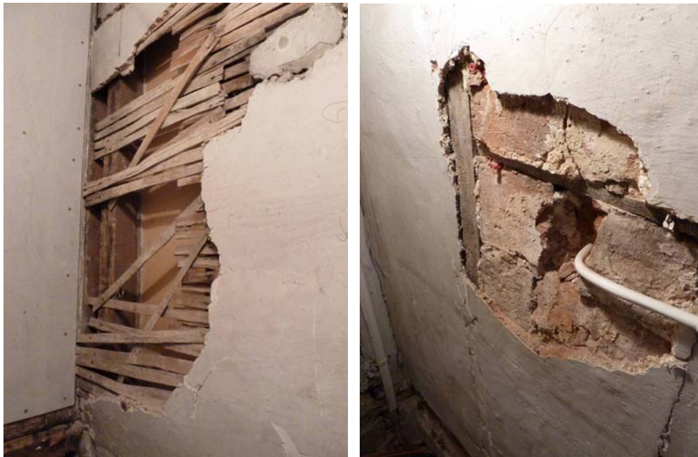
Stair to cellar – Left: Lath and plaster. Right: Brick infill
