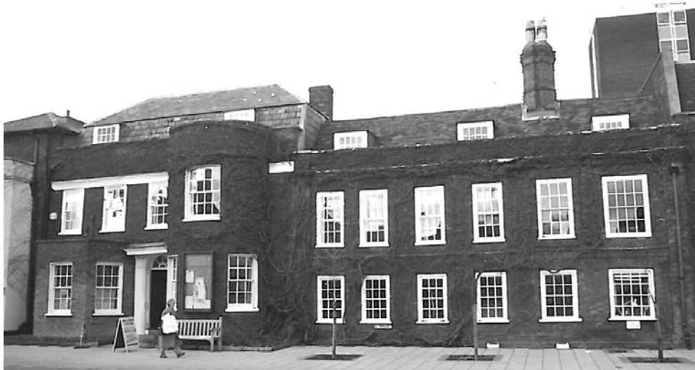
Shenfield Road elevation – Top: 2008
