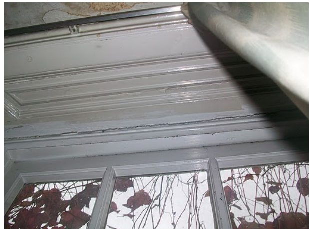
Left: Room 4 – Three (of four) sashes – Binding joist probably supported by RSJ
