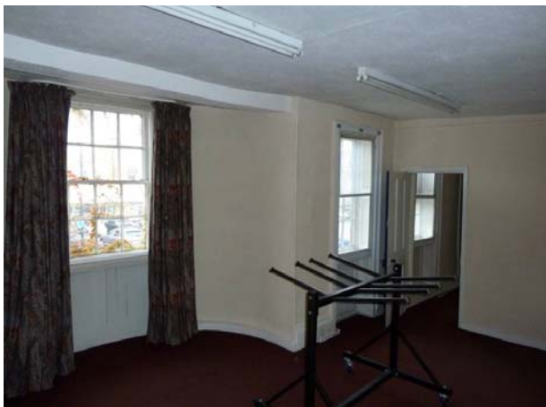
Left: Room 3 – One sash in curved bay – One sash adjacent to bay with secondary glazing
